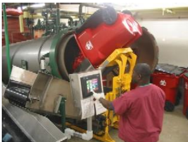
Loading medical waste into the Rotoclave ®
